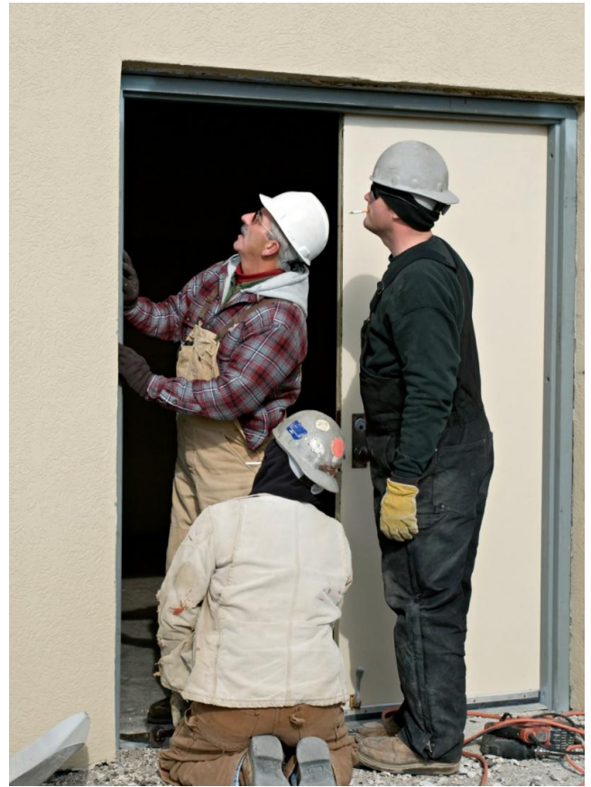
Figure 1.1. Workers in the construction trades face many hazards. The industry has a high rate of injuries and even deaths. The man on the right is making things even worse by smoking on the job, which is against the rules. Smoking is a serious fire hazard on the job and makes his health risk even worse. (Photograph ©dreamstime.)
