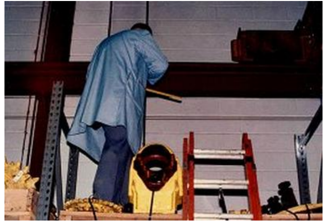
Figure 2.2. This worker is completely unprotected, up on an elevated platform without guard rails. The ladder is also too short and there is clutter on the walkway that could easily cause him to trip and fall to the concrete floor below. If he falls on his head from this height, the brain damage that could result could be permanently disabling.
