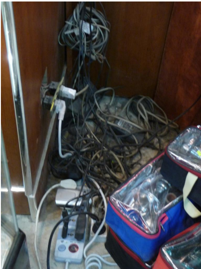
Figure 2.3. Too many electrical plugs in too few outlets. These electrical cords and outlets at a store in Egypt are dangerously overloaded. The wall outlet is poorly wired. This situation is likely to cause a fire.
